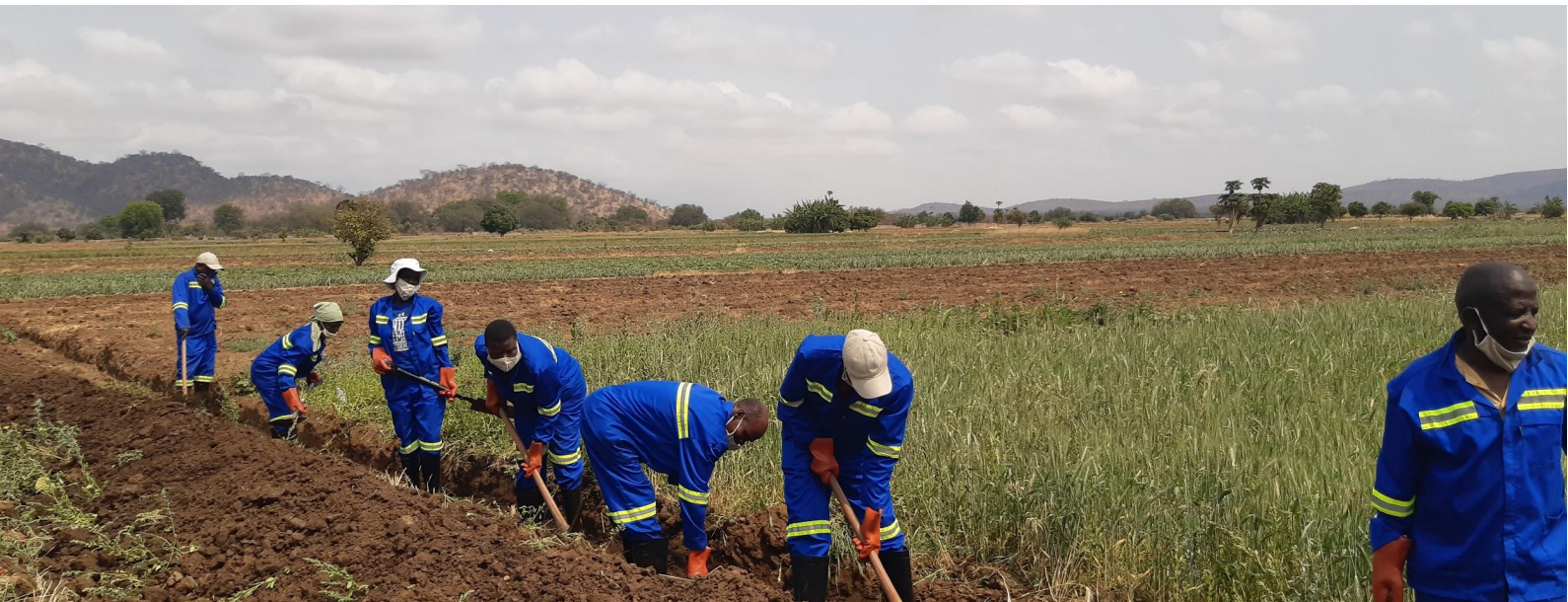
Community workers digging tail end drains at Gudyanga Irrigation Scheme @2020
