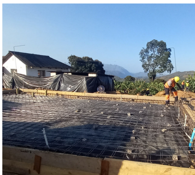
Steel fixing in progress at Mutsvangwa Maternal Health Center
