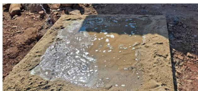
Scrubber plinth under curing
