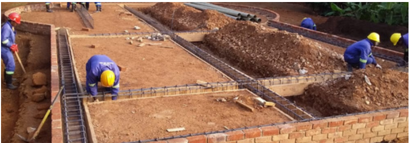
Laying of ground beam reinforcement at Hode Primary School
