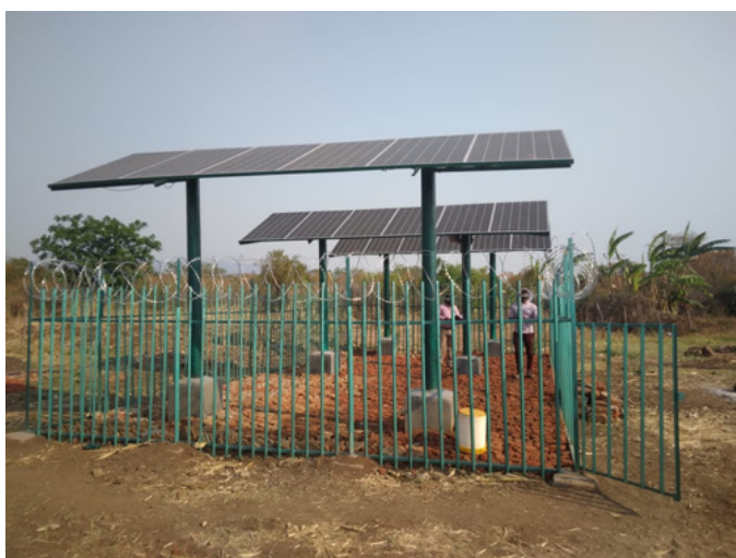
Solar powered water schemes being constructed under ZIRP
