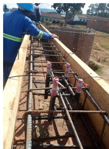
Above left: Steel fixing to grade 3 block Centre: Preparation for concrete pouring on ring beam Right: Concrete beam on Grade 1 block
