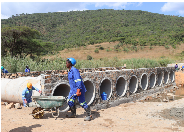
Culvert works at Ruwedza Road in Chimanimani
