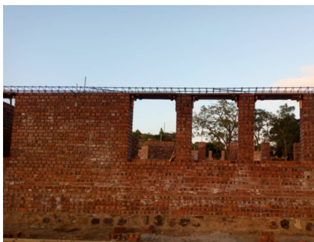
Above left: Steel fixing to grade 3 block Centre: Preparation for concrete pouring on ring beam Right: Concrete beam on Grade 1 block
