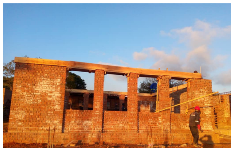
Above left: Progress on toilet block at Kushinga Primary School Right: Shuttering to grade 2 block in preparation to pour concrete for ring beam
