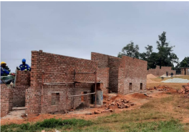
Works on superstructure at Jopa Market
