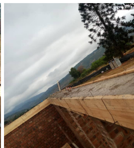
Above left: Steel fixing to grade 3 block Centre: Preparation for concrete pouring on ring beam Right: Concrete beam on Grade 1 block
