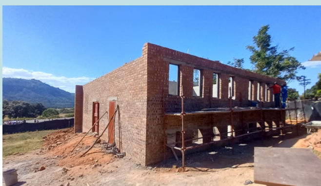
Works on superstructure at Jopa Market
