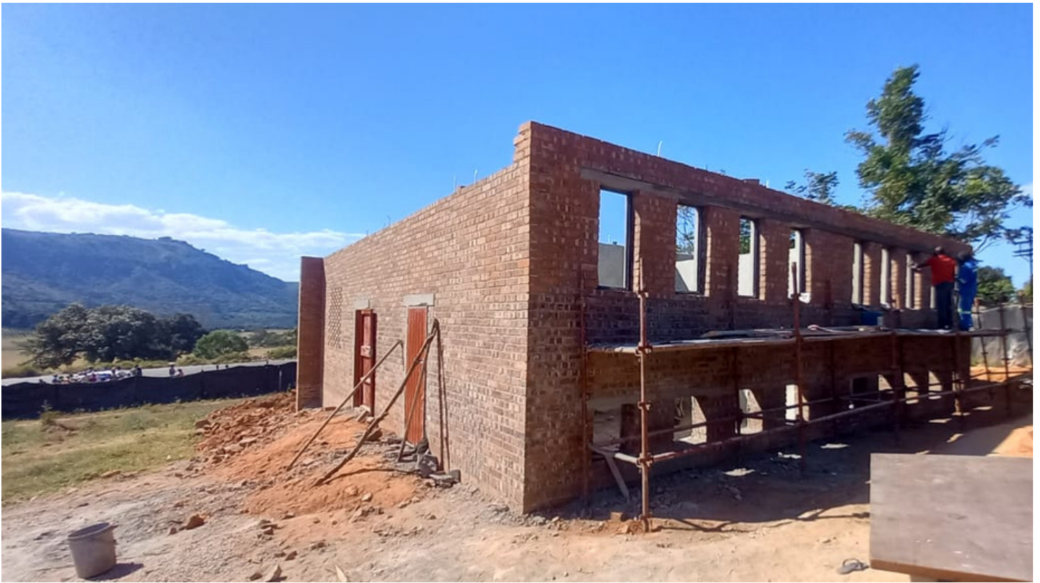
Progress at the new Jopa Market
