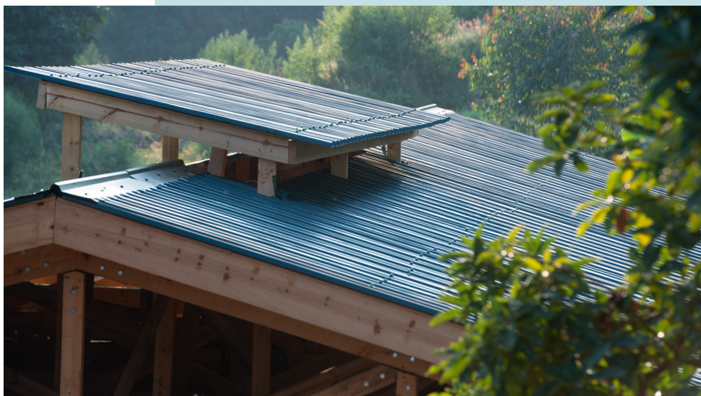
Above: roof of the Hode School toilet block.
