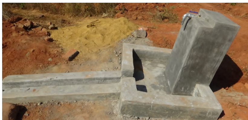
Right: A completed waterpoint.
